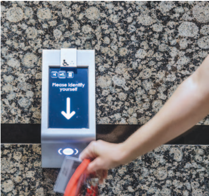
Photo left: PORT card readers are used to offer personalized Schindler elevator service for tenants while providing customizable access control within Three Lakeway. Photo right: Polished stone on the walls and floor of the elevator bank in the lobby of Three Lakeway creates a dramatic entrance.
